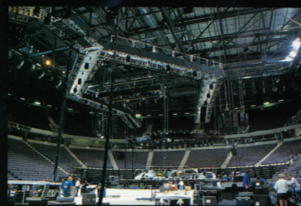
The catwalk in position, suspended above the arena
